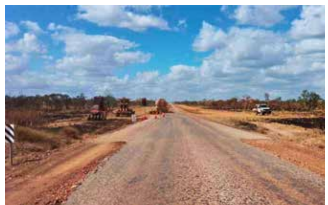
On-site images of Roper Highway Shoulder Rehabilitation.
